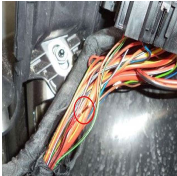
Figure 5: Clean wire stripped back at J1 splice point.
