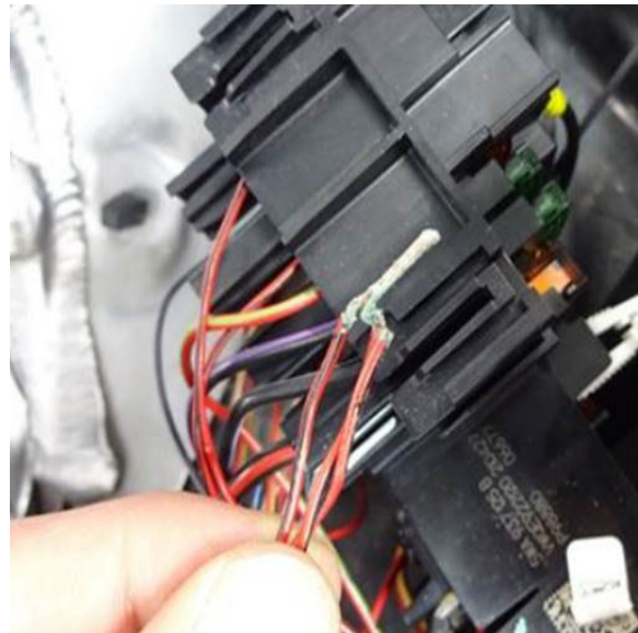
Figure 2: Corrosion found at splice point J1.
