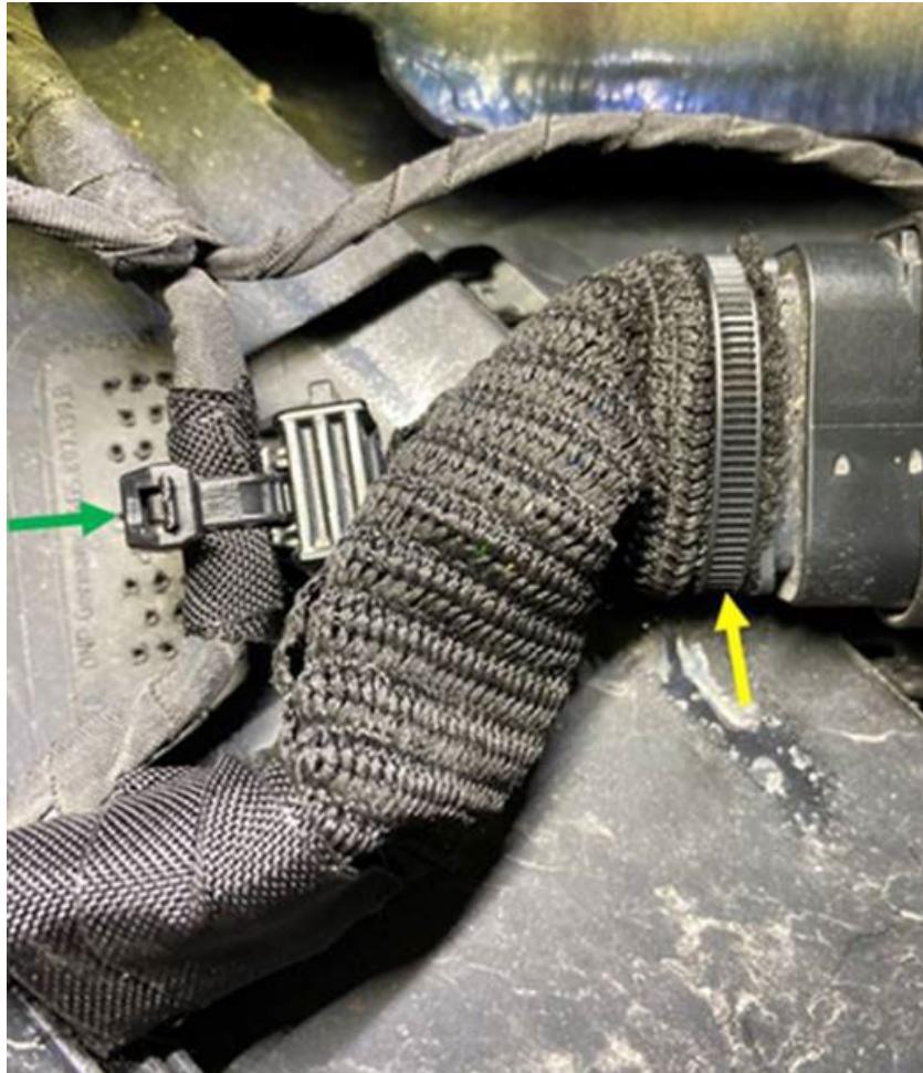
Figure 3: Completed repair of harness connection T14mx
