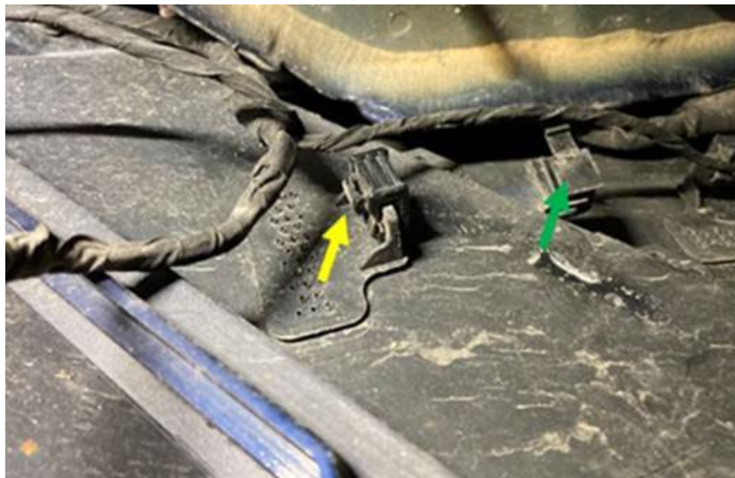
Figure 2: Cable ties to be removed
