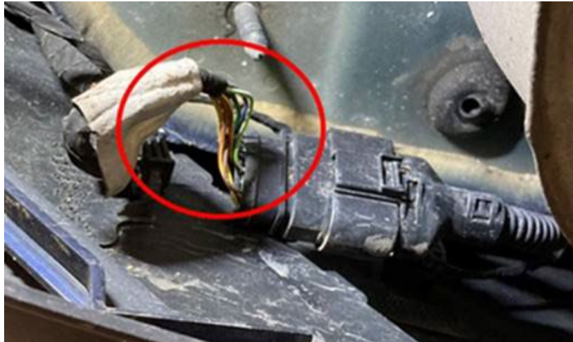
Figure 1: Inspection point of TSFHL
