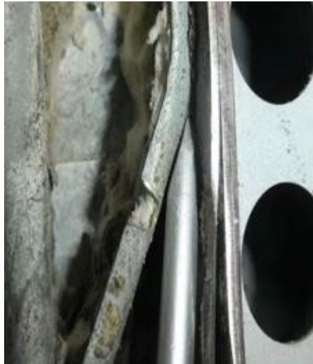
Figure 15. Correct engagement of the chisel end of the steel rod.
