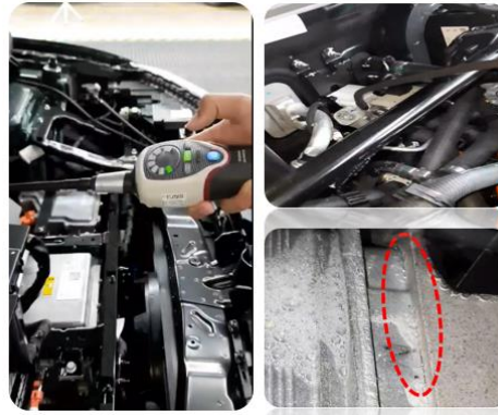
Leakage confirmed with Sniffer and Air bubble
