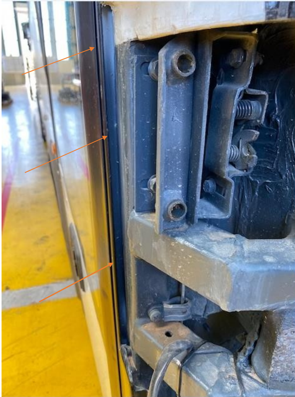
Figure.3. The front view of the area where the sealer is applied
