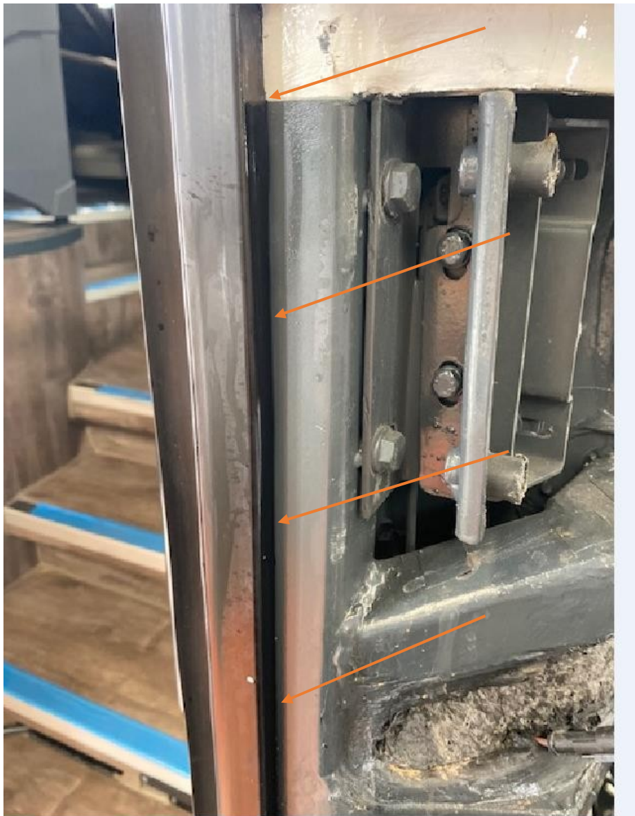
Figure.2. The side view of area where the sealer is applied
