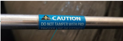
C CAUTION DO NOT TAMPER WITH PRD TRIGGER LINE OR FITTINGS, p/n 10602158 REV A
