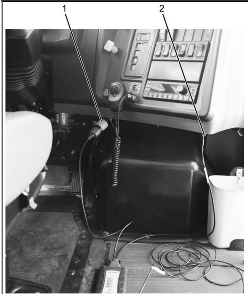
Figure #1: Y Cable Installation Bus
