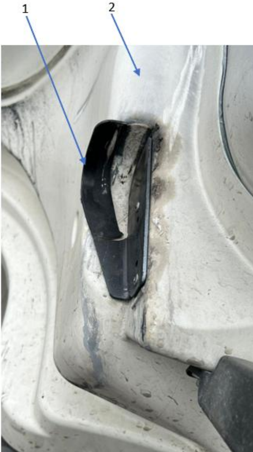
Figure 1. Hood Bracker Guide Broken
