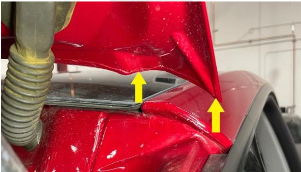
Figure 23 – Example of liftgate assembly seam
