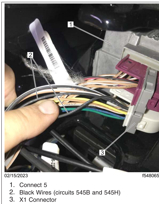
Fig. 20, Locating Existing Circuits 545B and 545H Connecting to Connect 5
