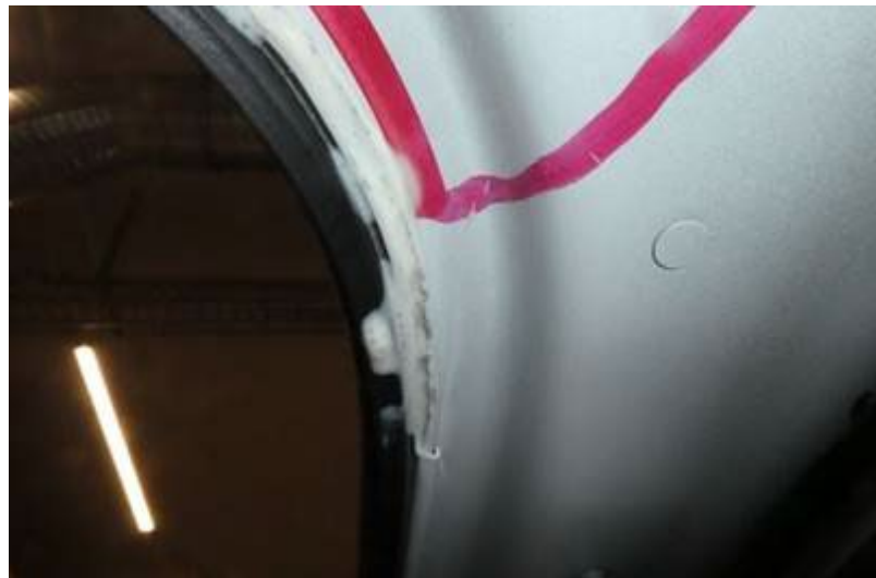
Figure 9. Gap created filled with Cavity Wax.
