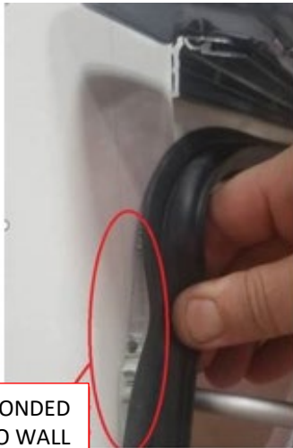
FIGURE 9 PROPER BUTYL ADHESION TO WALL
