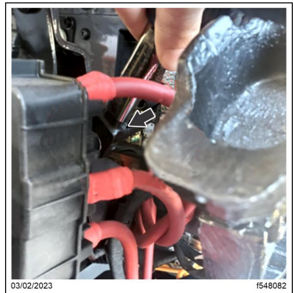
Fig. 8, Tightening the Front Fuses
