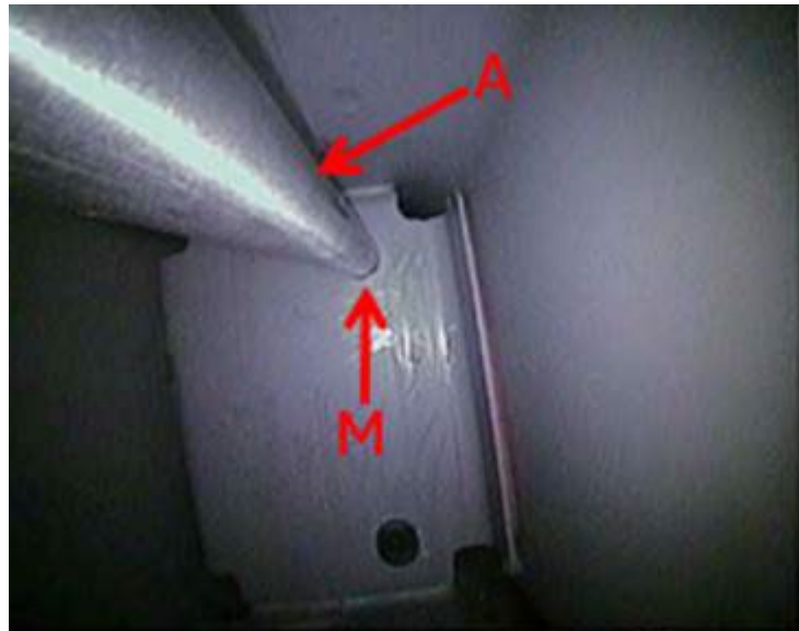
Figure 20. Feeding the steel rod through the reinforcement plate.
