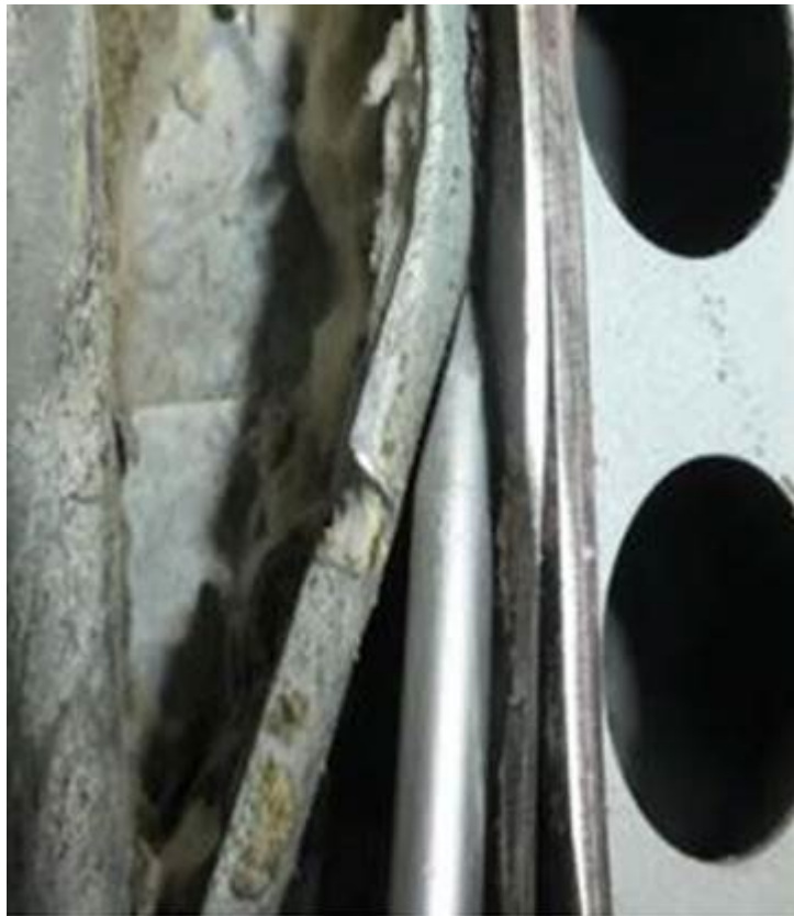
Figure 23. The chisel end of the steel rod properly engaged with the reinforcement plate.
