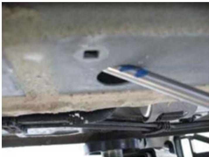
Figure 25. Marking the steel rod.
