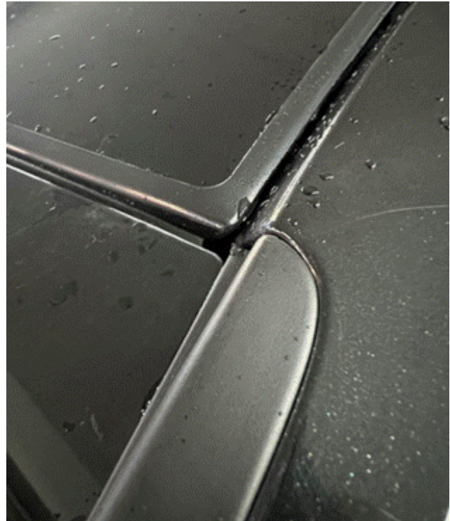
Figure 15. Drip rail trim reinstalled showing the desired opening for proper water drainage.
