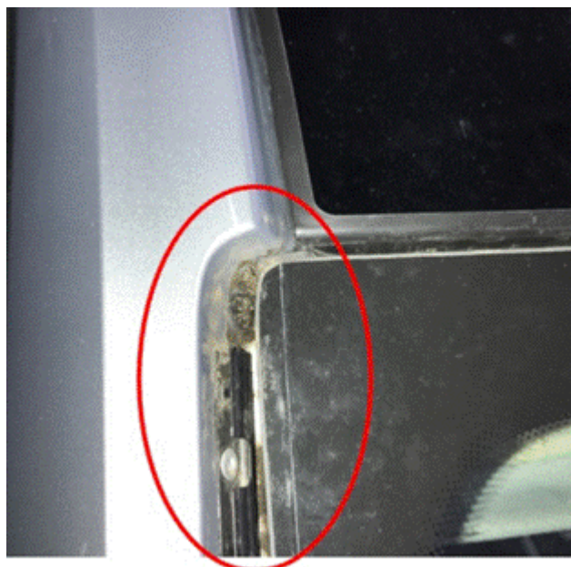
Figure 7. Drip rail trim removed exposing the accumulation of dirt and debris.
