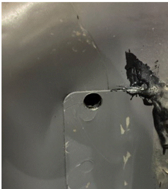
Figure 6. Completed drilled 6.5 mm hole in the cross panel section.
