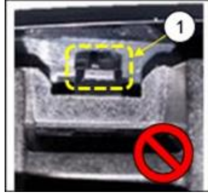
DETAIL A (1) Damaged tab
