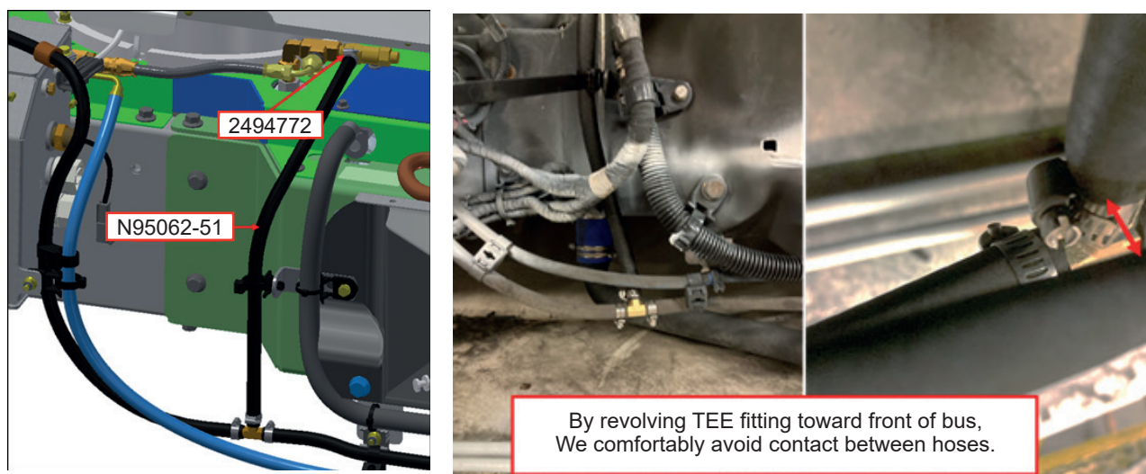
Figure 9 - Installation of Relief Valve Hose
