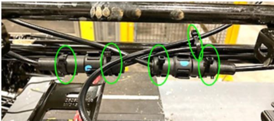
Fig. 6 Cut Off Zip Ties
