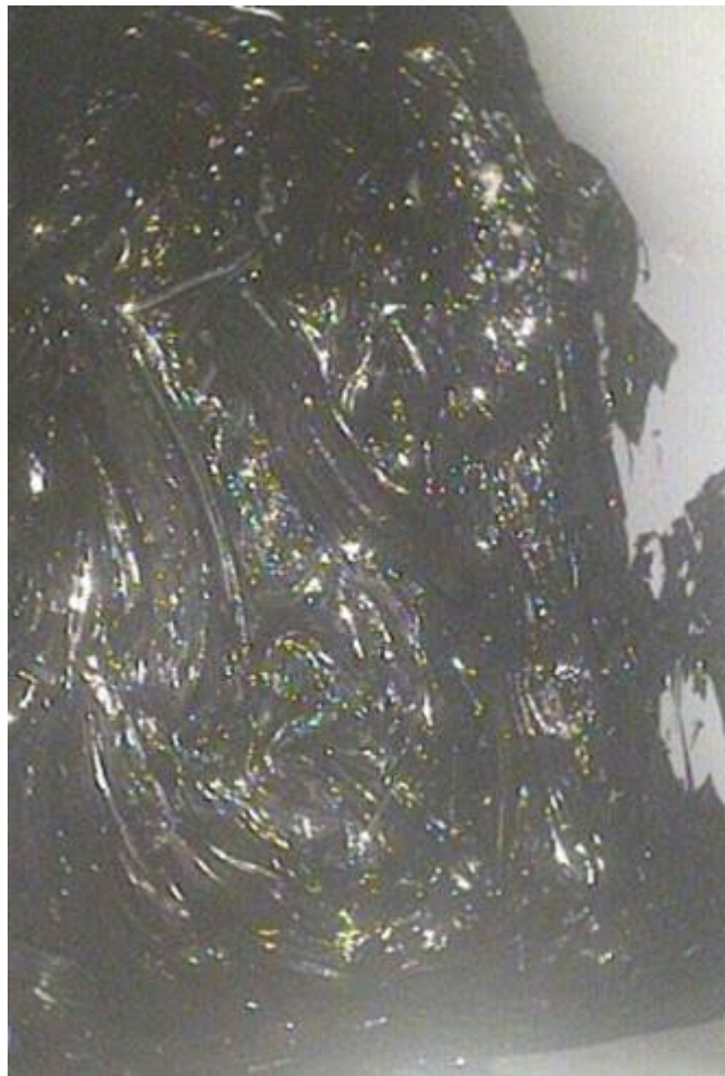
Figure 13. Sealer is completely applied and distributed.
