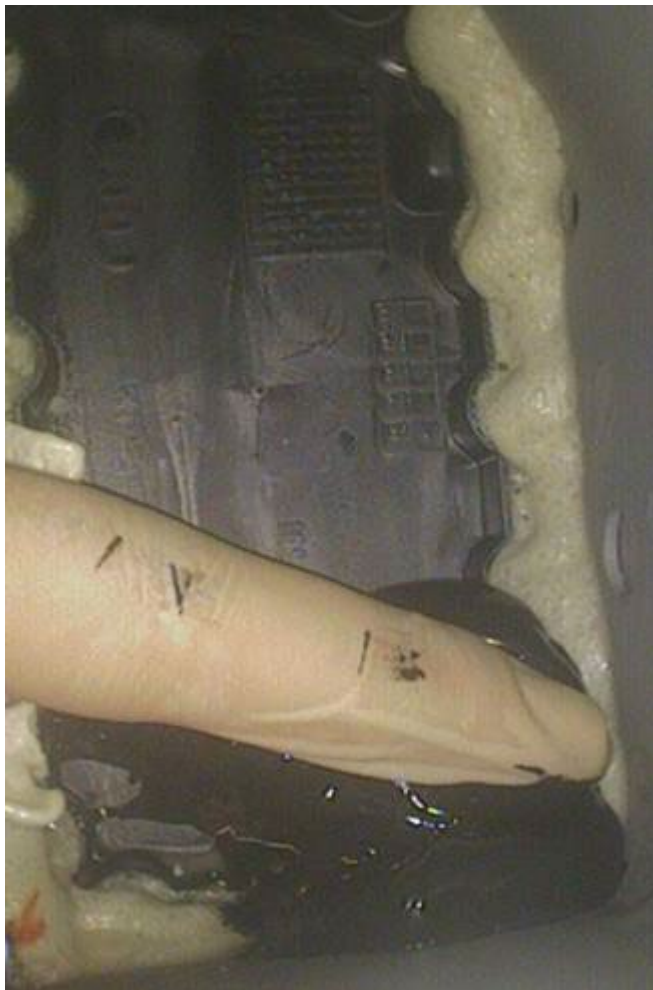
Figure 10. Distributing sealer over the web plate.
