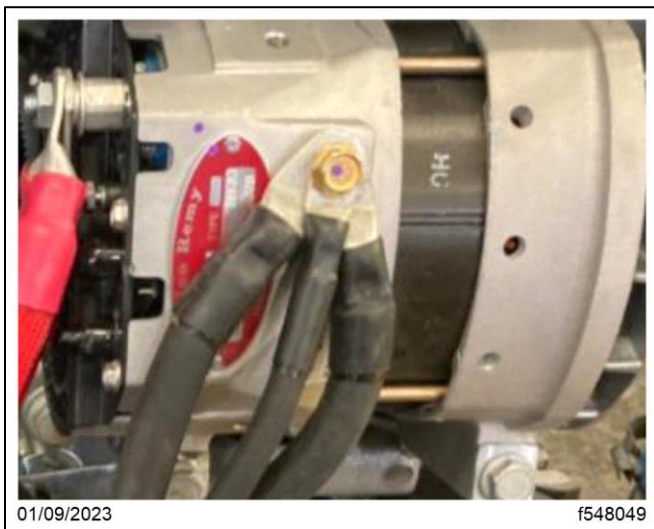
Fig. 1, Ground Cables Mounted on the Alternator
