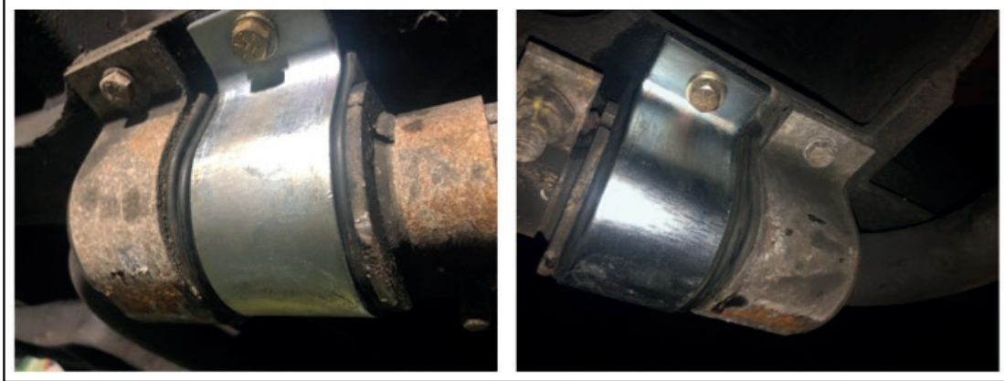
Figure 30 - Installation of Bracket and Hardware
