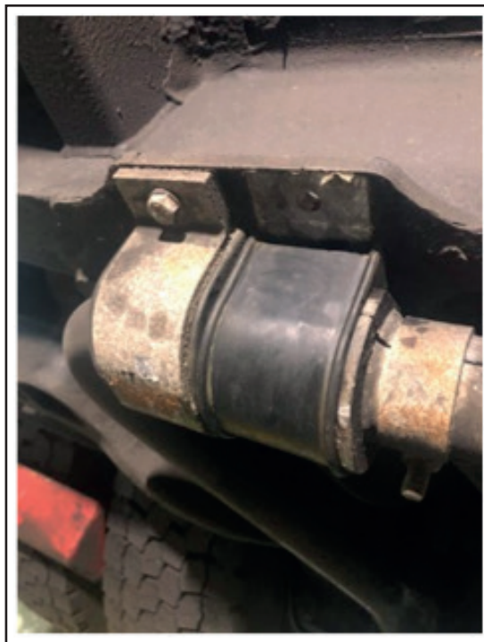
Figure 29 - Installation of New Bushing
