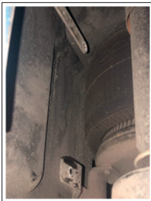
Figure 20 - Removal of Leveling Valve
