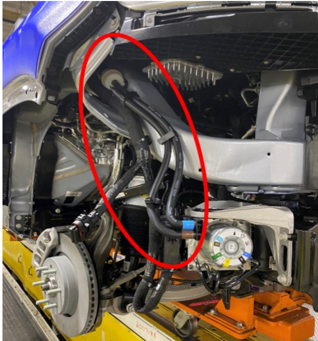
Fig. 1 Vent Hose and (ASCM) Connection
