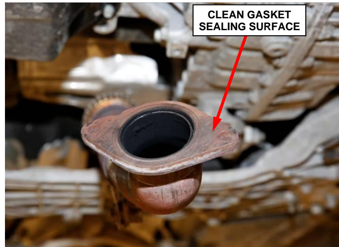
Figure 29 – Crossunder Pipe Flange
