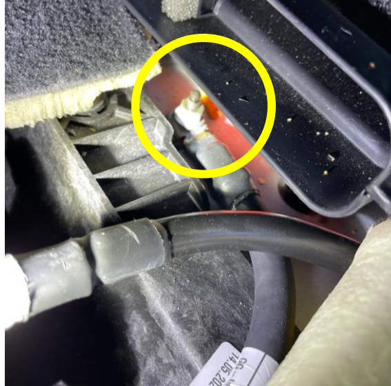
Battery (-) Ground Stud G919A
