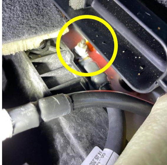
Battery (-) Ground Stud G919A
