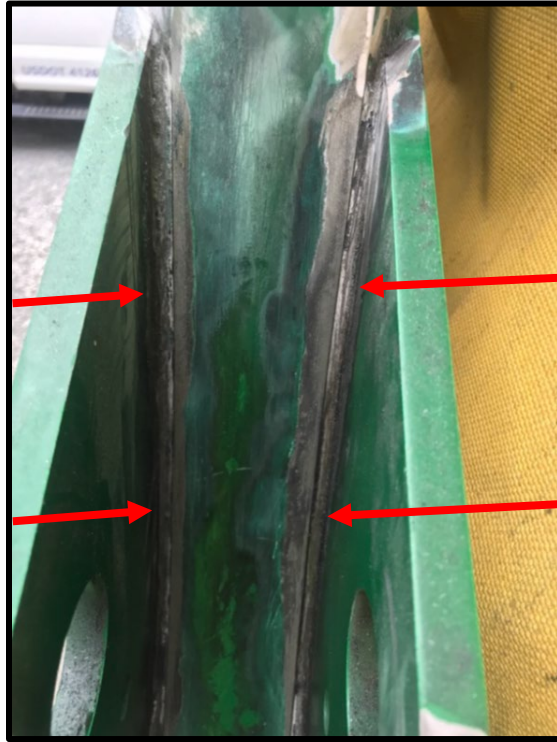
Figure 7 Cleaned Weld Area
