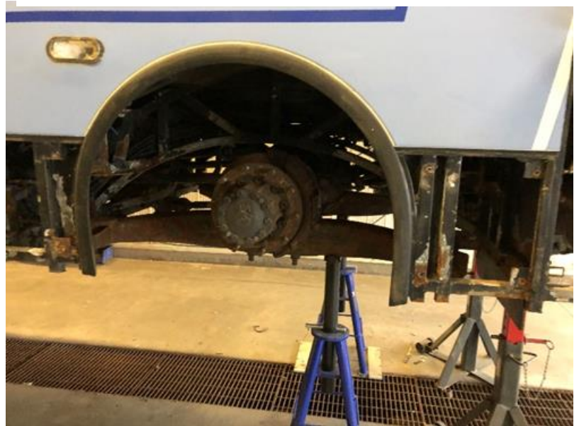
Axle and structure supported
