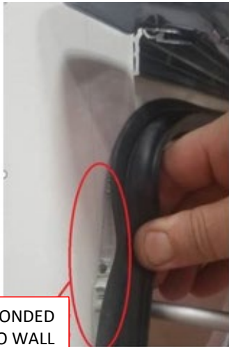
FIGURE 9 PROPER BUTYL ADHESION TO WALL
