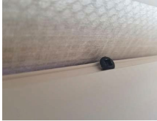
FIGURE 3 – PROPERLY INSTALLED WALL CLIP SECUREMENT SCREW
