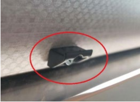
FIGURE 2 – PROPERLY INSTALLED WALL CLIP
