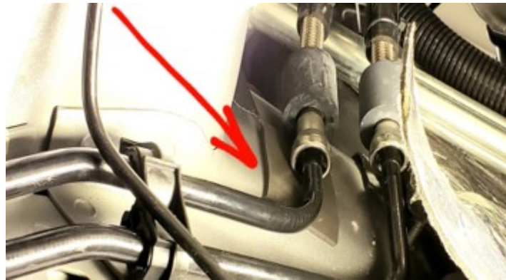
Fig. 10 Foam Patch Installed
