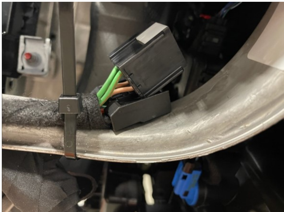
Fig. 2 Securing the Loose Wire Harness
