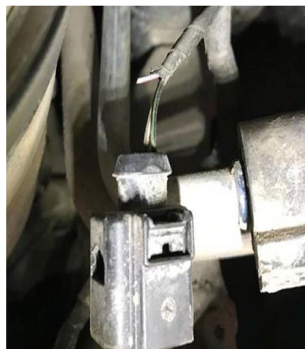
Figure 1. N280 control wire damaged at T3r connection
