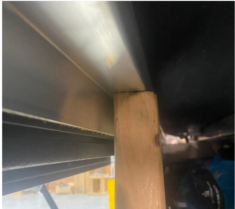
Photo example 3. Alignment of 2x4 supporting upper deck.
