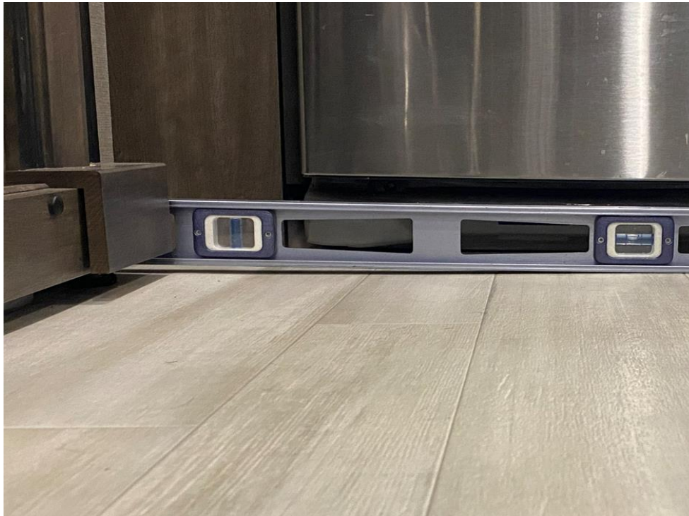
Photo example 1. Inspecting the floor for sag.
