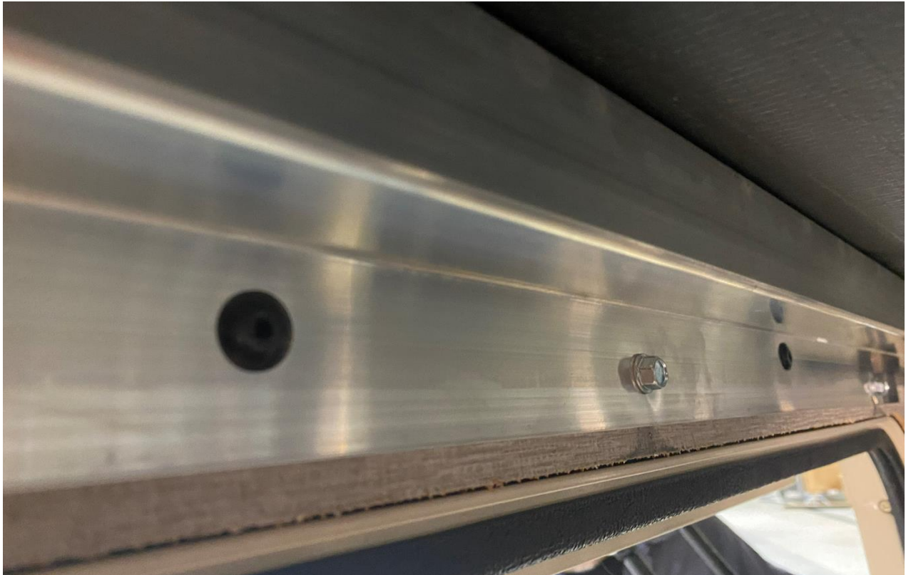
Photo example 4. Repaired P-tube with screws and rivets installed.
