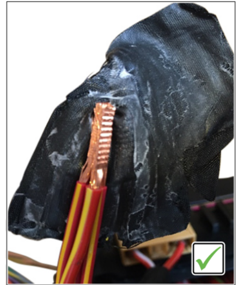
Example of splice connection OK
