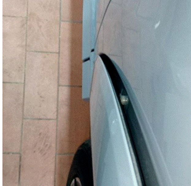
Figure 1. The front wheel arch trim is not flush to the fender surface.
