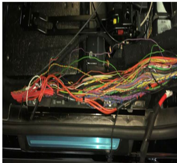
Figure 2: Driver side door sill area, open harness to expose splice points.
