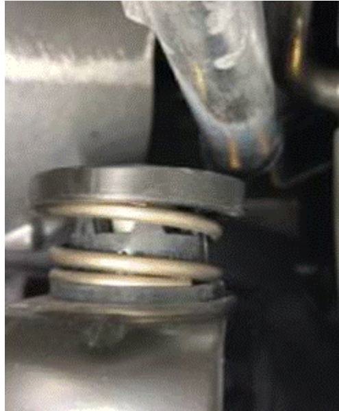
Figure 10. Correctly seated compressor isolator / spring assembly.
