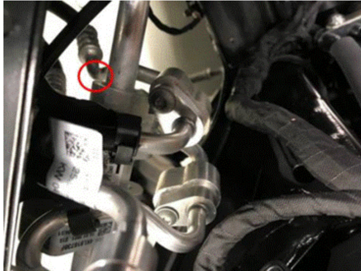
Figure 8. Point of contact between coaxial refrigerant line and the refrigerant line containing the service port.
