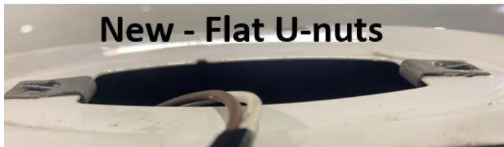
Images show the difference between the old and the new U-nut
