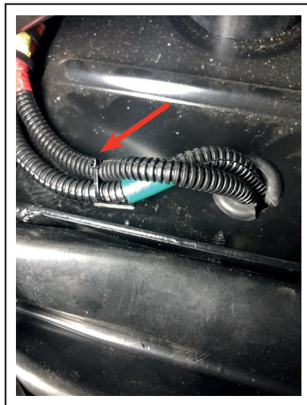
Figure 9 - Installation of Tie Mount to Harness
