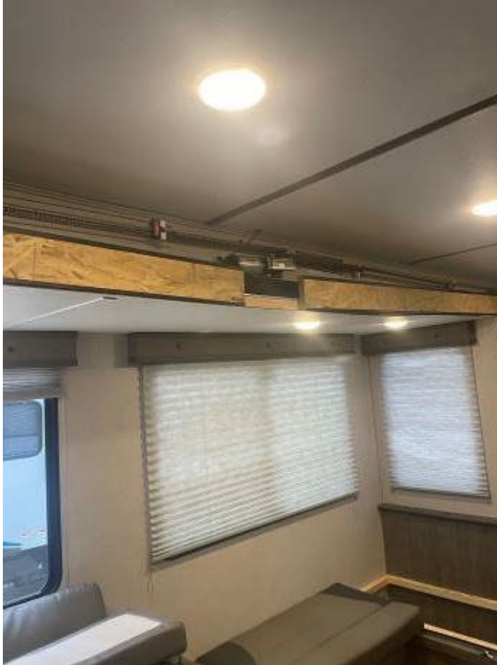
CURRENT HEADER INSTALLED
