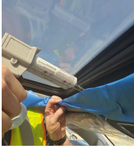
Fig. 8 Applying Glue
