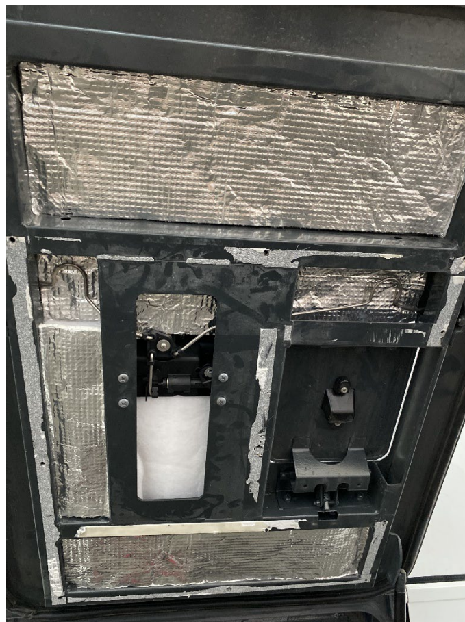
Figure.7 The final image of the application of insulation
