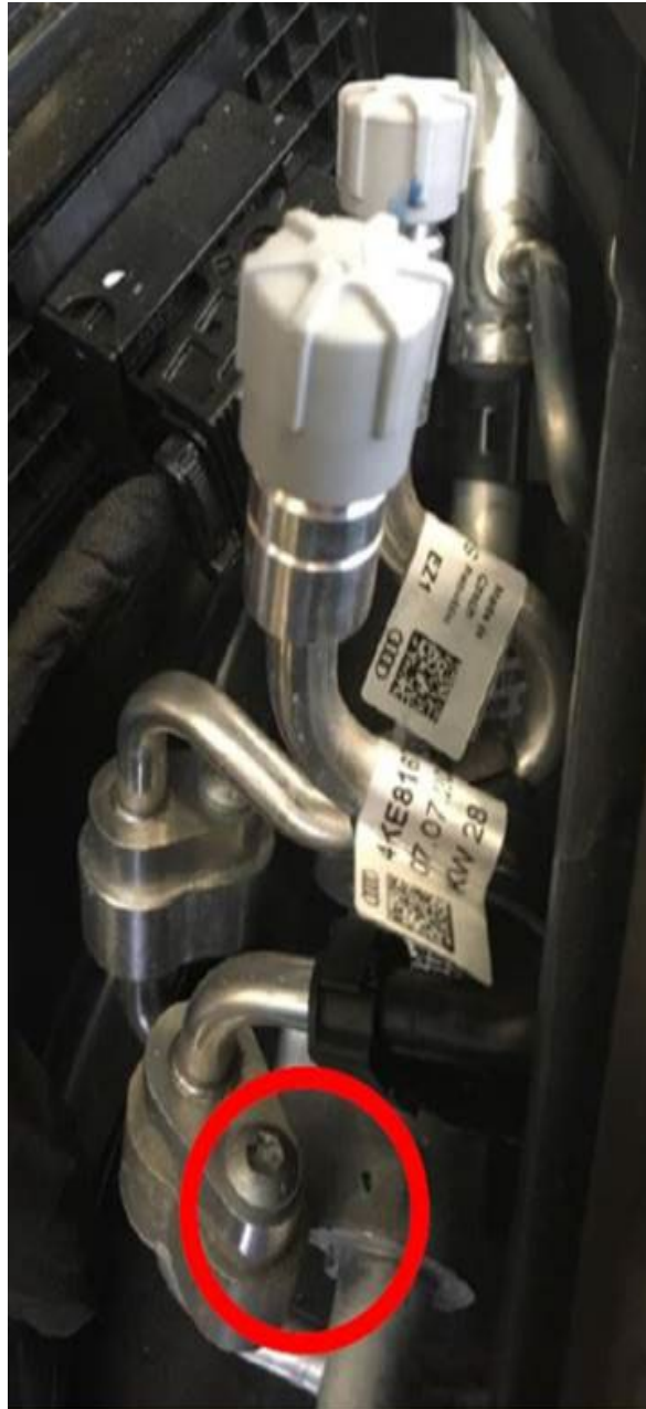
Figure 3. The refrigerant lines are making contact.
