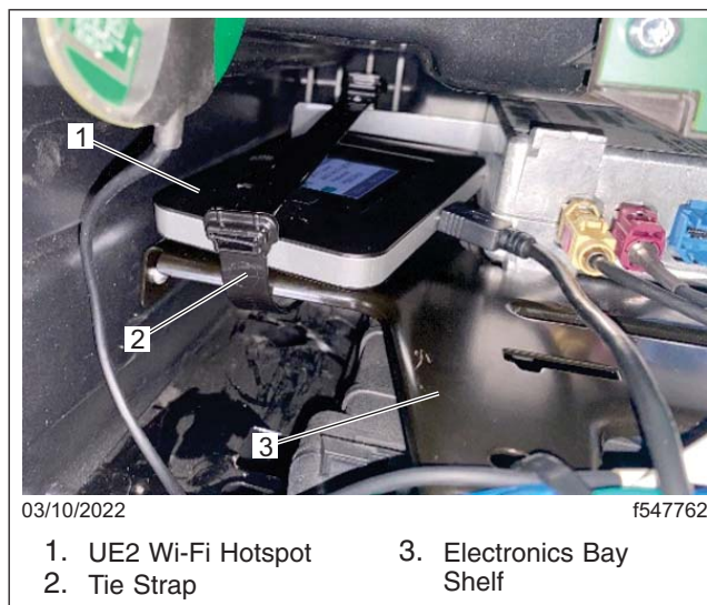
Fig. 42, UE2 Wi-Fi Hotspot Device Installed
