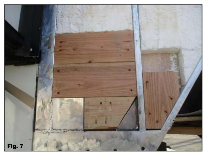
Pre drill using 3/16" drill bit through 2X6 LCI steel tube (upper deck), add screws Horizontal through triple hollow wood stuffed sidewall tubes into center of steel tube adding (4) 1/4"-20X3" screws. See Figures 8 and 9.
