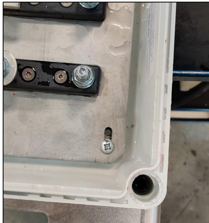
Figure 9: Example of drilled hole through plastic and metal plate
