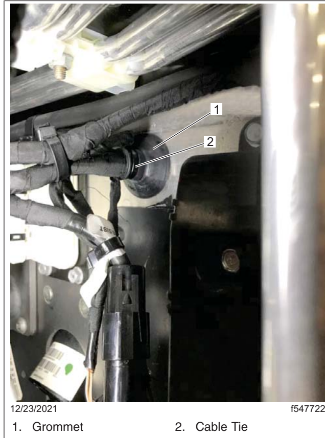
Fig. 12, Firewall Grommet and Cable Tie
