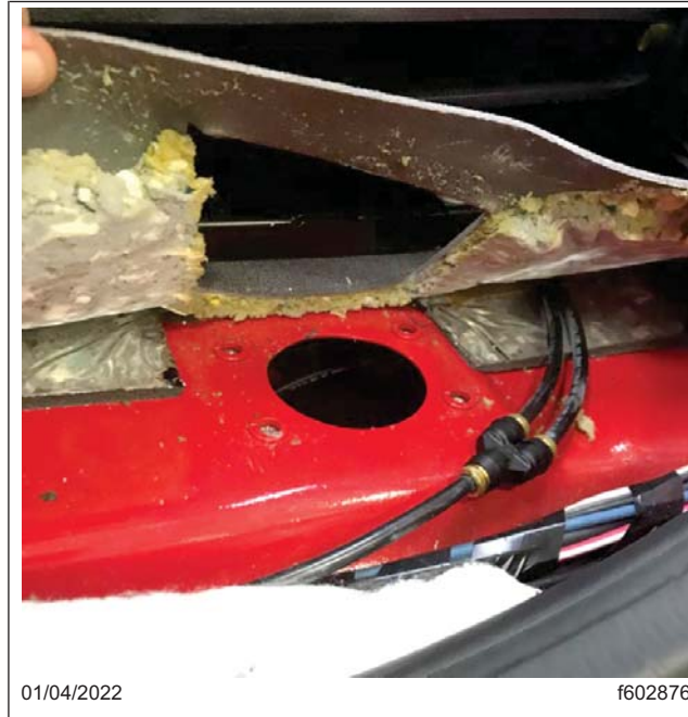
Fig. 21, Holes Drilled for Battery Load Disconnect Switch
