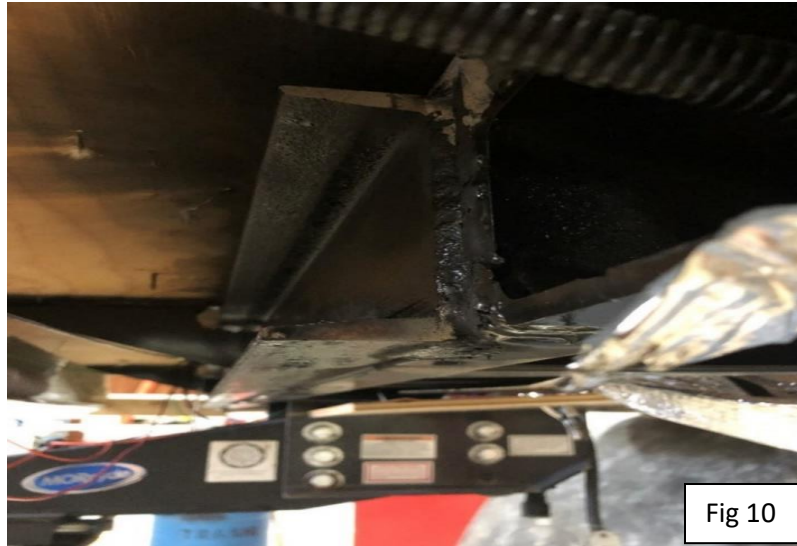
Figure 10 shows the structural C-channel welded
