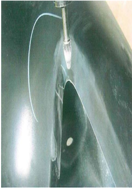
Grind crack with deburring tool
