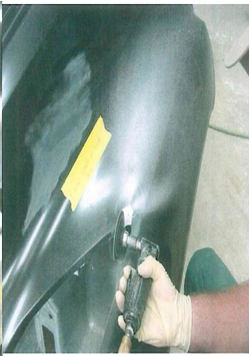
Grind area around crack with 24 grit disc
